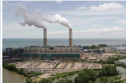
MONROE POWER PLANT
