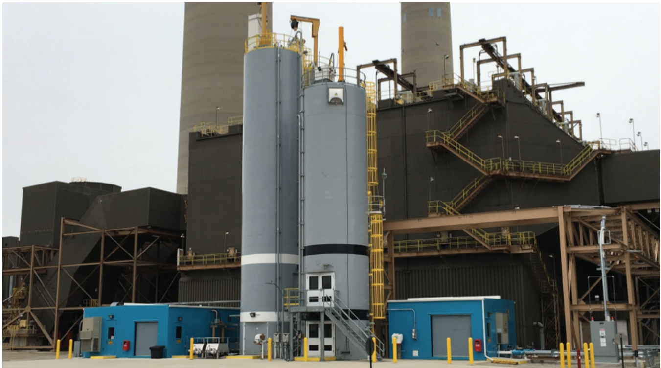
Photo: DTEE Belle River Power Plant MATS control equipment
