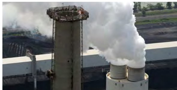
WATER VAPOR IS RELEASED FROM ONE OF TWO NEW STACKS AT THE MONROE POWER PLANT AS WORKERS DECONSTRUCT ONE OF THE PLANT'S ORIGINAL STACKS
